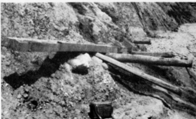
Section of railway exposed by cliff fall
